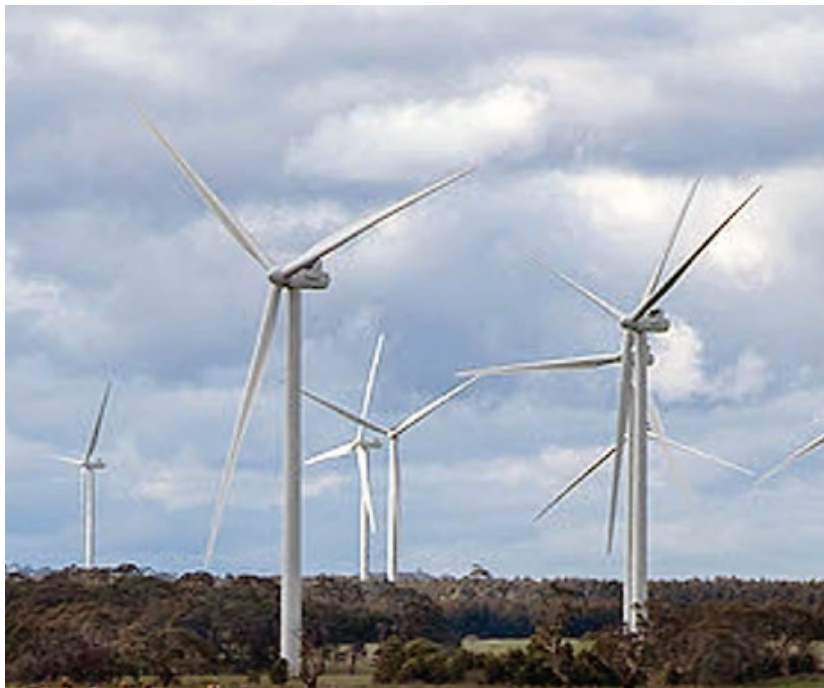
Vestas has received an order for the supply and installation of 46 wind turbines for CS Energy's Lotus Creek wind farm in Central Queensland. (Courtesy: Vestas)
