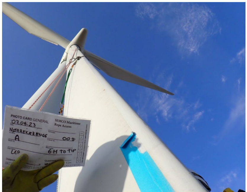
Figure 1: Leading edge protection of wind turbine blade using polymeric technology. (Courtesy: Belzona).
