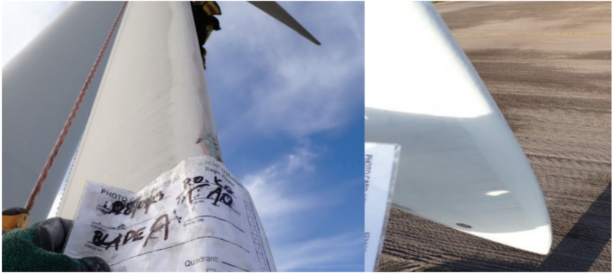
Figure 4: Leading edge repaired and protected with Belzona 5711 and Belzona 5721. (Courtesy: Belzona)
