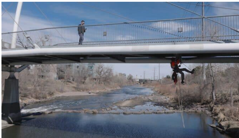
Figure 1: Construction worker placing IoT sensors [7].
