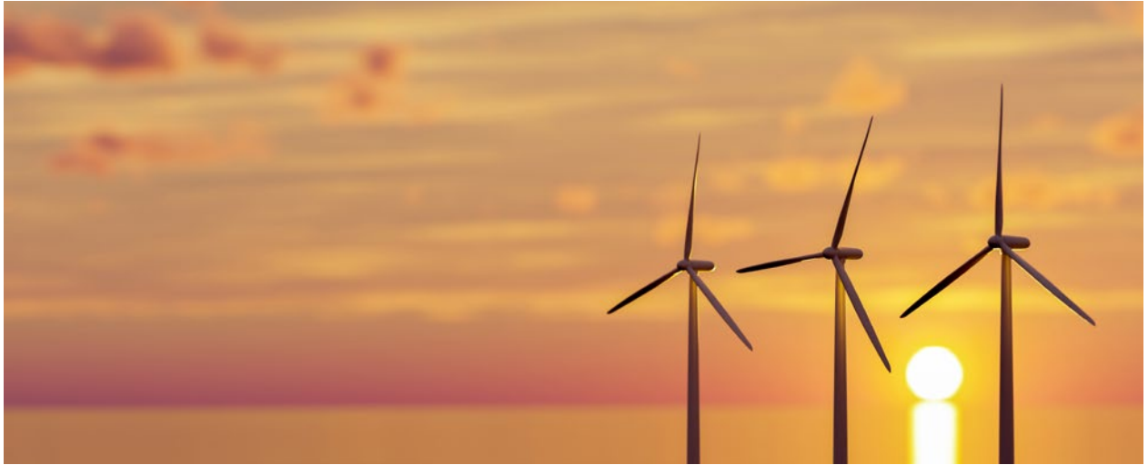
Digital twin technology has the potential to increase the lifespan of floating offshore wind turbines. (Courtesy: Shutterstock)
