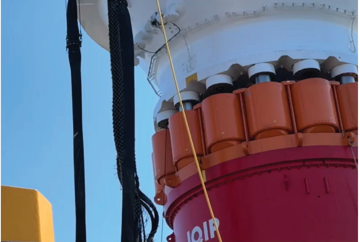
EQ-Piling helps to achieve noise-compliant monopile installation. (Courtesy: IQIP)
