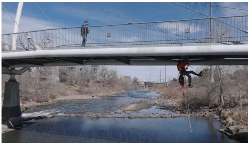
Figure 1: Construction worker placing IoT sensors [7].
