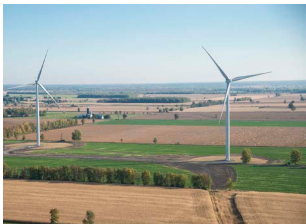
The windiest areas of the country aren't necessarily the areas with the best access to transmission. (Courtesy: Siemens Gamesa)
