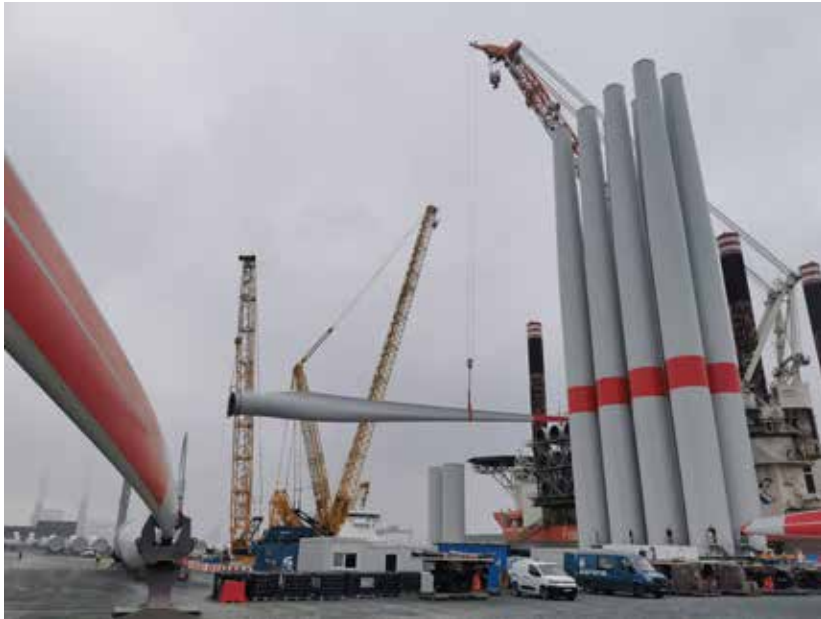
The first wind farm in Brittany has been completed. (Courtesy: Sarens)
