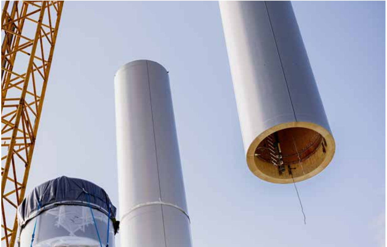
A wooden tower is a third lighter than a comparable steel one and, as a result, is easier to transport. (Courtesy: Modvion)
