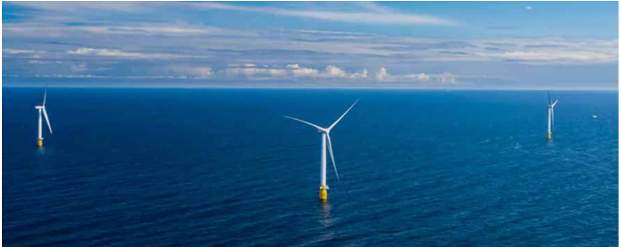
DNV recommends an offshore high-voltage direct current transmission network. (Courtesy: DNV)
