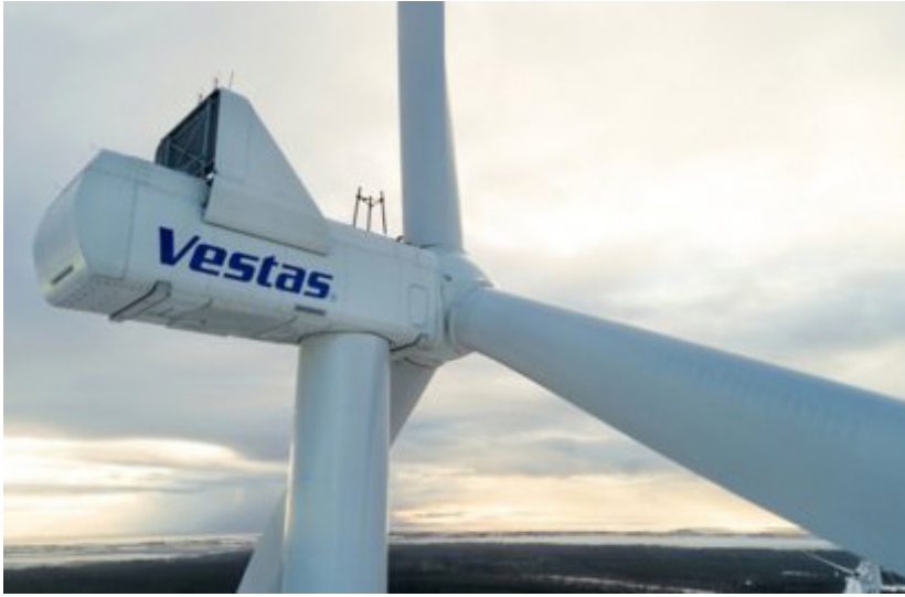
Commissioning for the Steelhead project is set for 2025. (Courtesy: Vestas)
