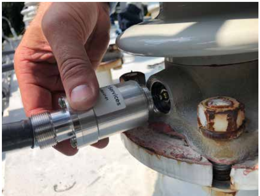
Precision engineered bushing sensors replace the grounding cover at the bushing base. (Courtesy: ZTZ Services International)
