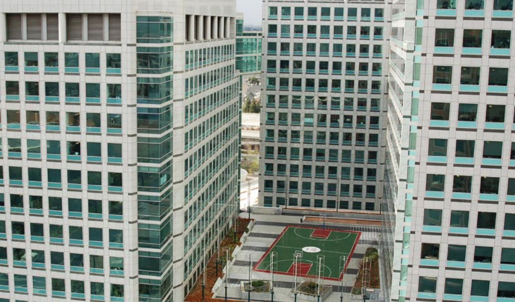
Fig. 2: Another view of the Windspire placements at Adobe headquarters.
