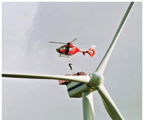
Fig. 3: Cranes and even helicopters must be chartered for some O&M work (gizmodo.com).
