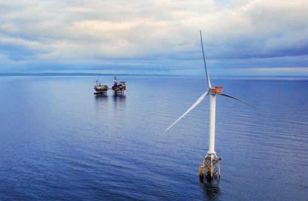
Fig. 2: The Beatrice Wind Farm Demonstrator Project off the East coast of Scotland.
