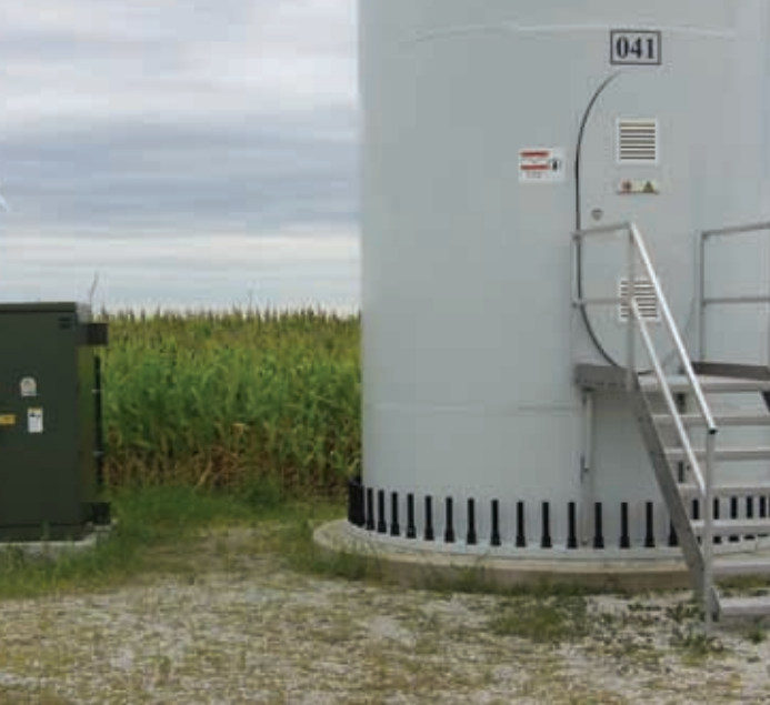
Fig. 4: Distribution setup transformer at base of a 1.5MW Acciona turbine.
