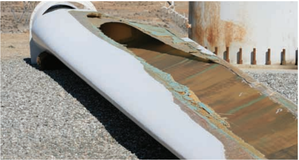
Fig. 1: Any tall structures, such as power poles or wind towers, are natural targets for lightning.
