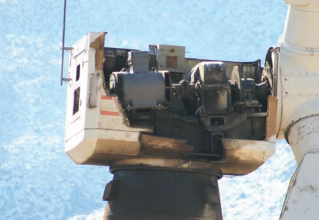
Fig. 3: The aftermath of a turbine fire.
