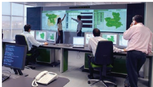
Fig. 2: Example of a Winergy CDS located in a central monitoring room.
