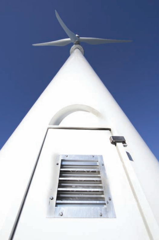
Fig. 3: KONE's compact Monospace elevator systems swoops visitors quickly and safely up the tower to the viewPod, beneath the nacelle.
