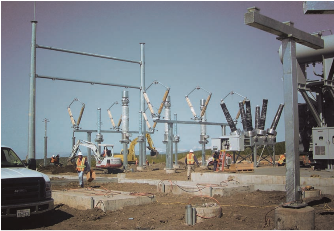
Fig. 2: The Hatched Ridge Wind Farm, under construction.
