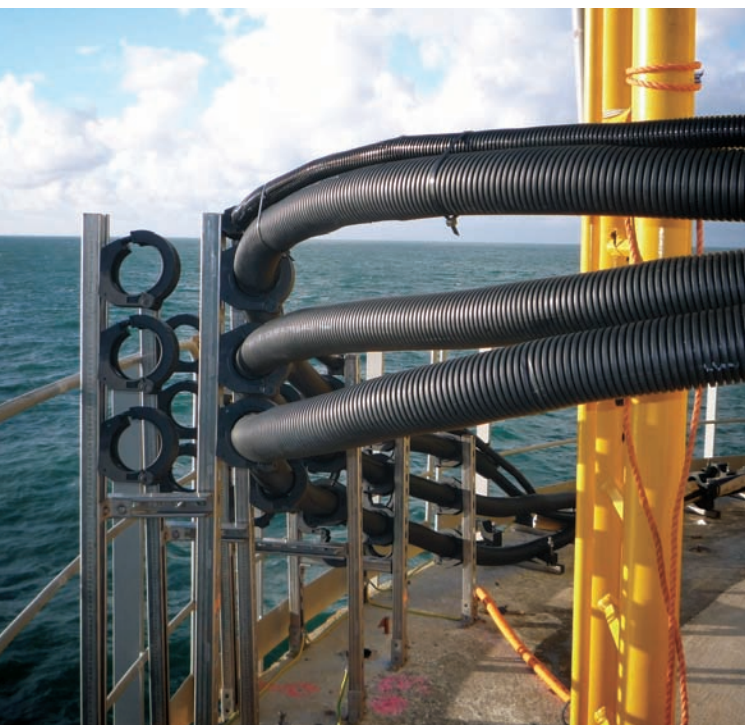
Fig. 1: PMA cable protection mounted on the deck of an offshore wind turbine can withstand intense, sustained exposure to the sun's ultraviolet rays.
