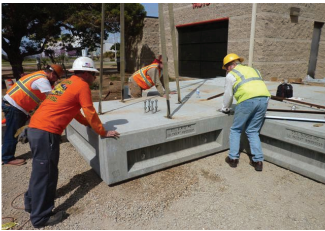
Fig. 2: Positioning Cell Blocks requires little equipment or manpower.
