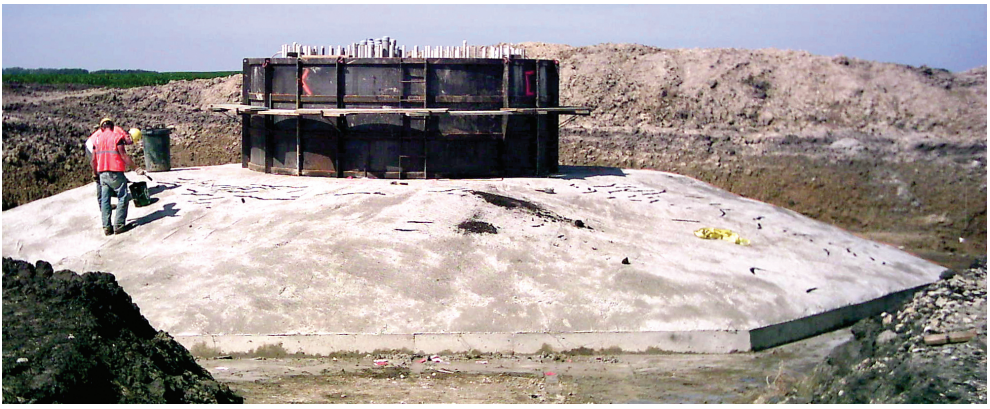
Fig. 3: Octagonal wind turbine base (preliminary work shown in fig. 2).
