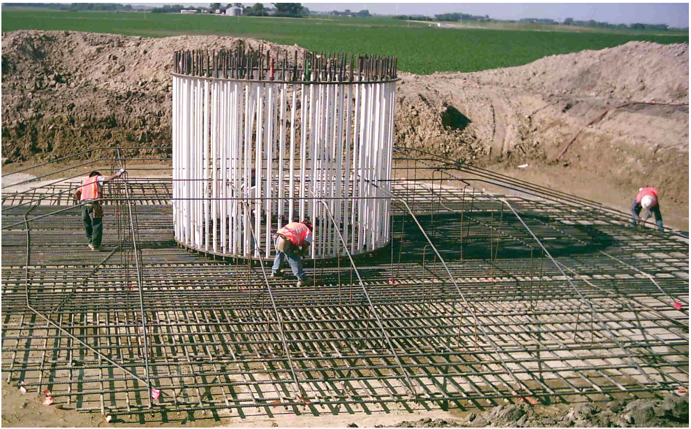
Fig. 2: Construction of a wind turbine base (see finished base in fig. 3).
