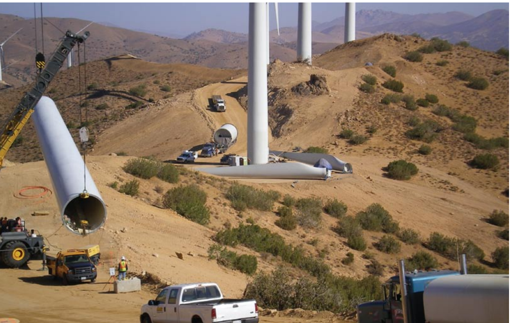
Fig. 2: Towers are erected at the Pine Tree Wind Project.
