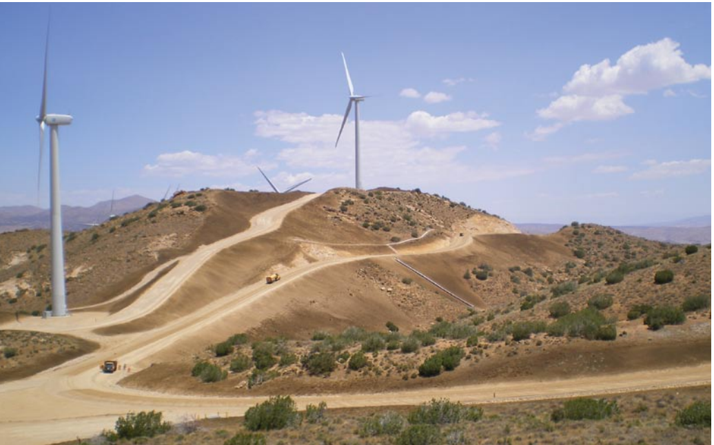
Fig. 1: A series of roads weaves through the Pine Tree Wind Project.
