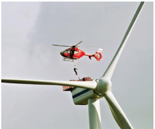
Fig. 3: Cranes and even helicopters must be chartered for some O&M work (gizmodo.com).
